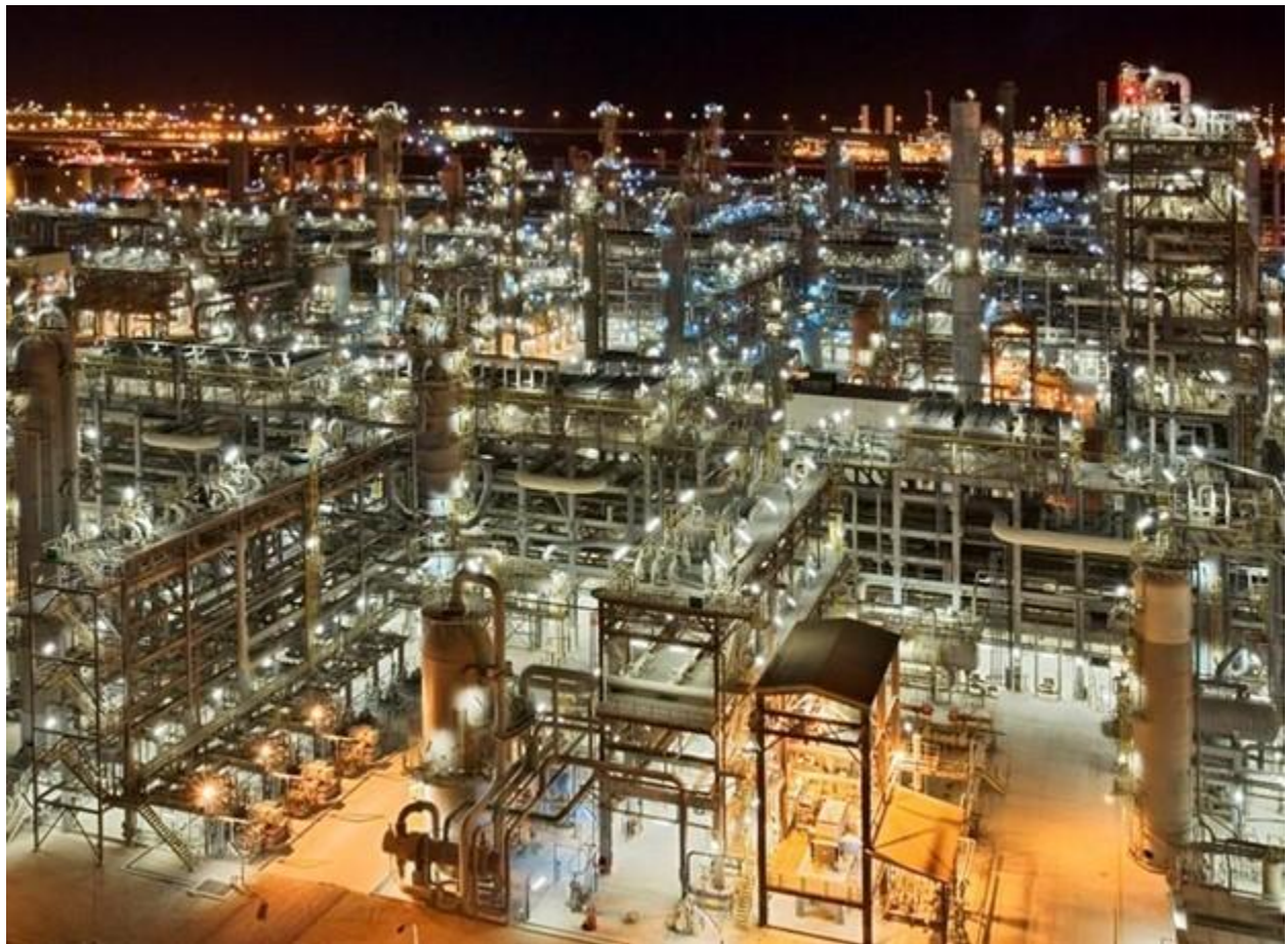
Ras Laffan Industrial City, pictured at night
